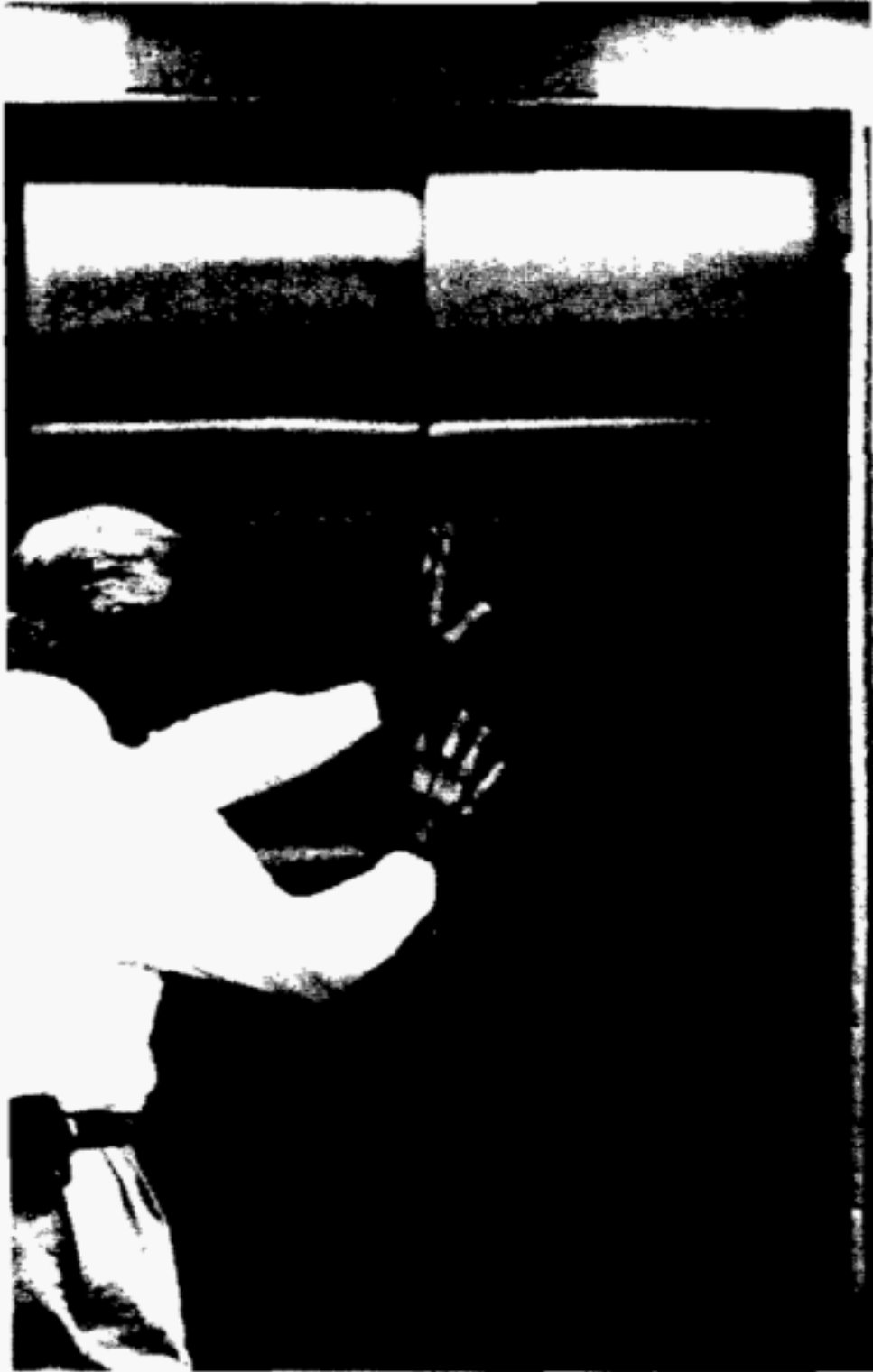
FIG. 1.3.4(c) OPENING OF CAR DOOR BY HAND (Not Possible on Some Elevators)
