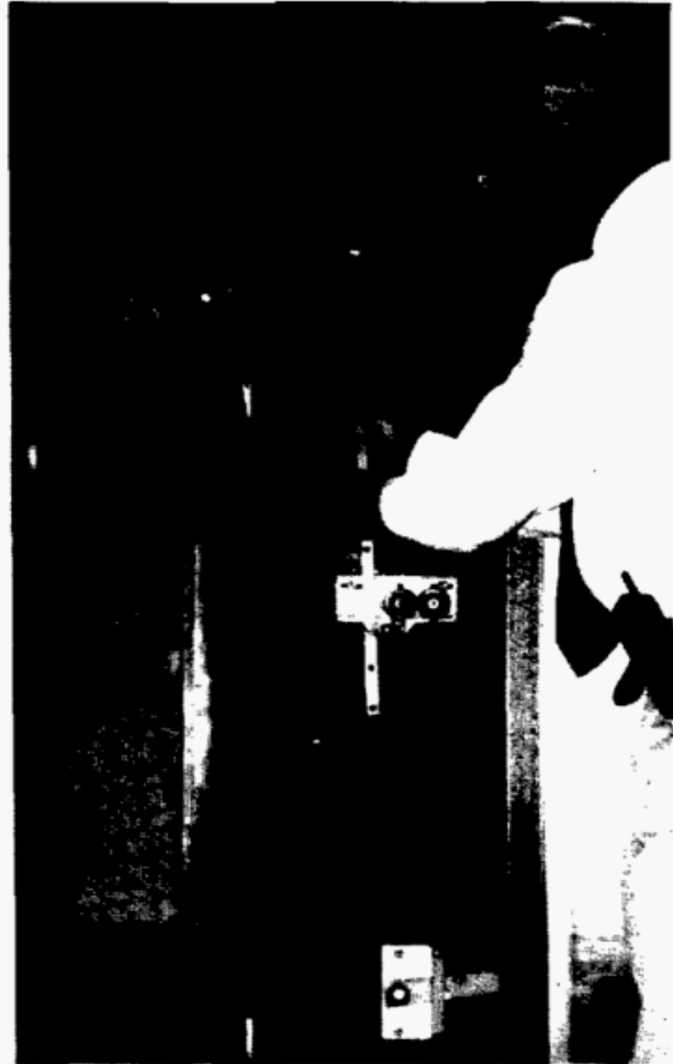
FIG. 1.3.4(d) OPENING HOISTWAY DOOR BY HAND (Not Possible on Some Elevators)
